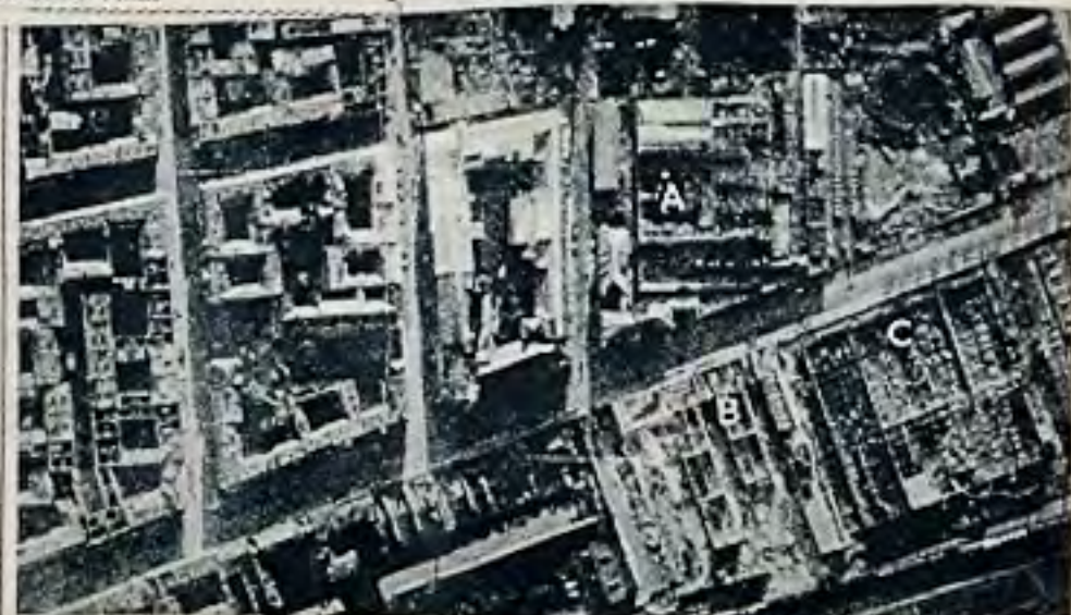
(A) THE RESULT OF HIGH EXPLOSIVE AND FIRE IN AN IRON FOUNDRY; (B) RADIO VALVE-MAKERS' PREMISES GUTTED; (C) LARGE BUILDINGS DESTROYED IN A WORKS MAKING TURBINE PARTS.
