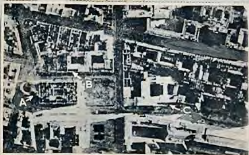
MORE DAMAGE IN THE CENTRE OF THE CAPITAL: (A) TOP FLOORS OF KAISERHOF HOTEL BURNED OUT; (B) TREASURY ROOF DAMAGED; (C) MINISTRY OF TRANSPORT AND STATE RAILWAYS DIRECTORATE
