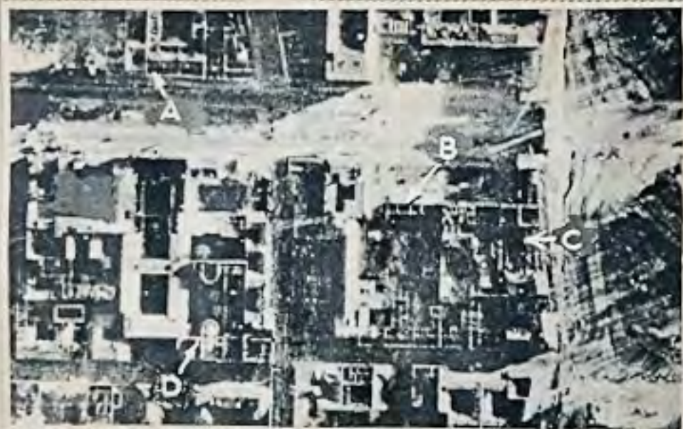
DAMAGE IN CENTRAL BERLIN: (A) MINISTRY OF EDUCATION DAMAGED BY FIRE; (B) FRENCH EMBASSY GUTTED; (C) MINISTRY OF ARMAMENT AND MUNITIONS GUTTED; (D) ARMY RECORDS OFFICE SEVERELY DAMAGED BY FIRE.
