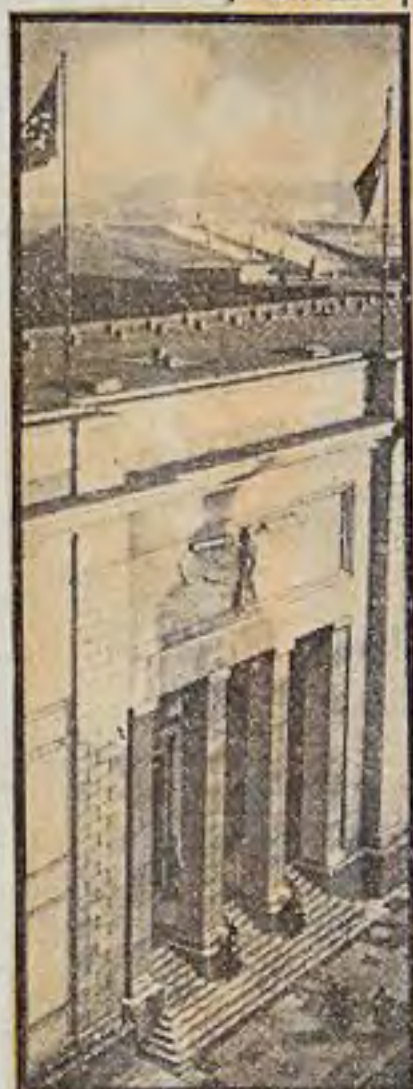
T HIS is Hitler's new Chancellery in Berlin, three-quarters of which is reported to have been destroyed in Sunday night's raid. It was completed in January 1939, and adjoins the old Chancellery. Its total street frontage was more than a quarter of a mile.
