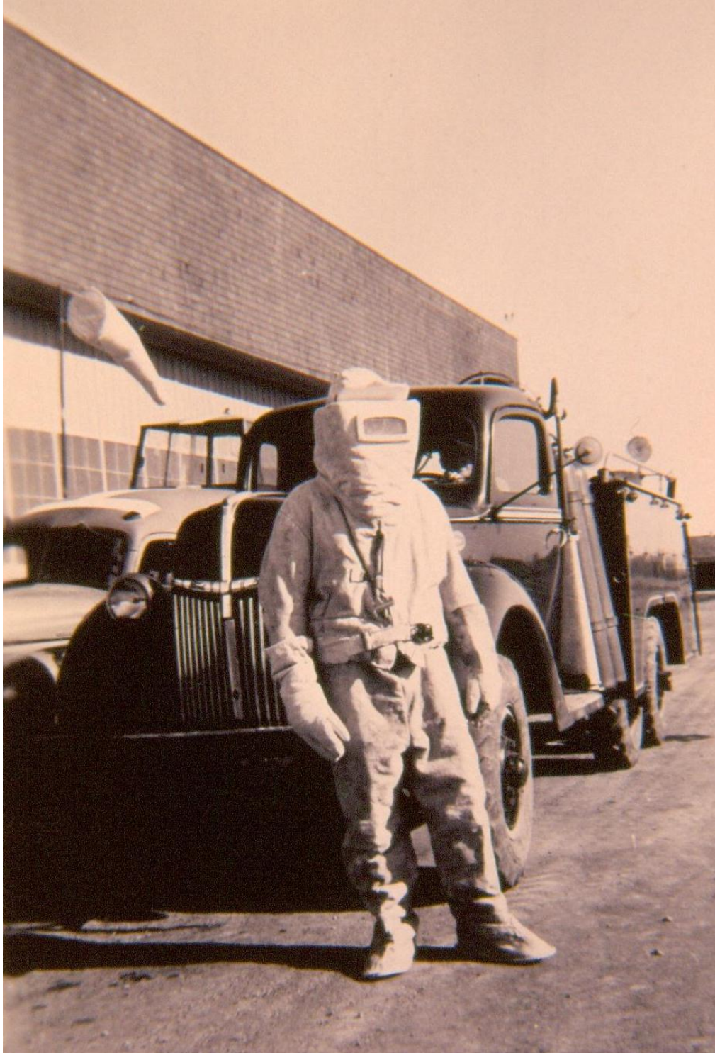
The RAF Airdrie Relief L.G. 1941 fire-crash truck, [Marmon-Herrington Ford 6X6] aircraft fire-rescue suit, and the mobile radio control tower truck, RCAF #31-129 with wind sock. The mobile radio tower vehicle was painted bright yellow, with complete top a bright red, with a large white letter "T" painted on roof for trainee pilots to see. Image taken in front of hangar doors, east side of building summer 1943.
