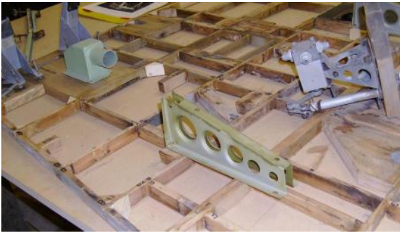
Components that will later be mounted to the floor are placed on top to make sure that all the necessary wood has been added back. There will be no opportunity to do so once the covering is added.
