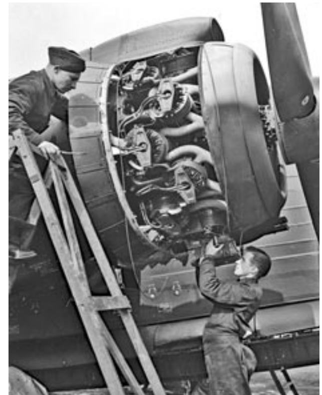
Servicing a Bristol Hercules radial engine
