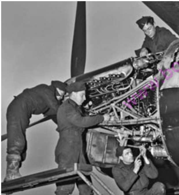
Aero-engine mechanics working on a Lancaster's Rolls-Royce Merlin engine
