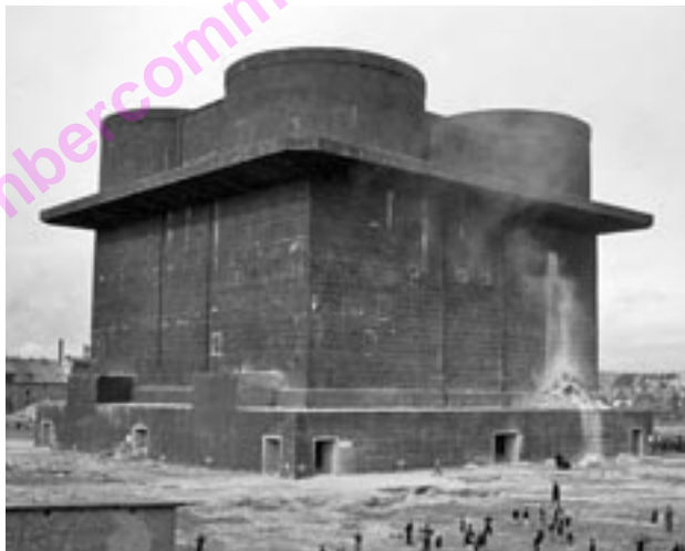
This post-war photo is of a huge 'flak tower, three of which were built in Berlin. As well as anti-aircraft guns, each included a radar installation with a radar dish which could be retracted behind a thick concrete and steel dome for protection.
