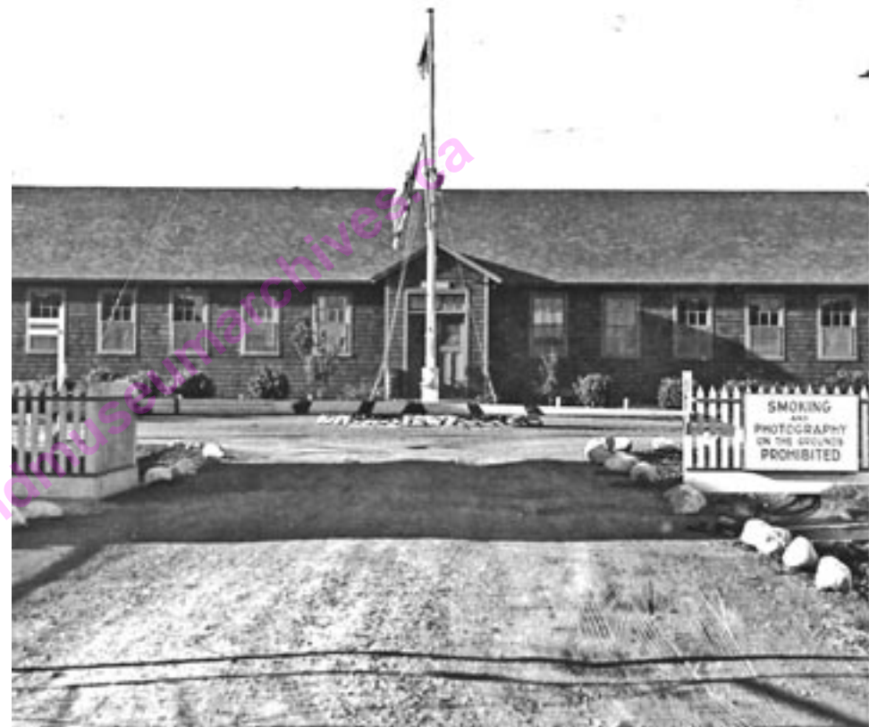
The main entrance to 5 Elementary Training School at High River, Alberta
