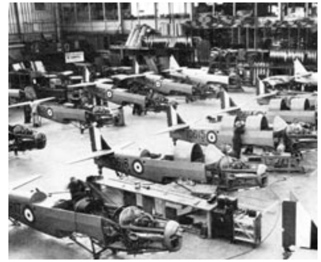
Building Cornell primary trainers at Fort Erie, Ontario. The Fleet Cornells eventually replaced the De Havilland Tiger Moth and Fleet Finch bi-planes at Elementary Flying Training Schools.
